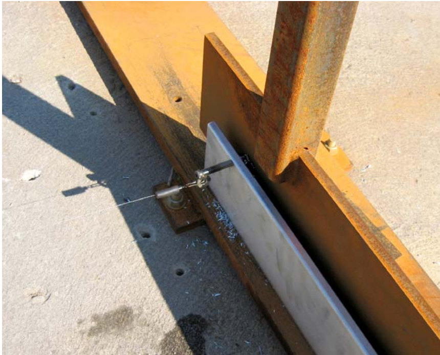
Fig. 7 - A close-up view of the deflection measurement point on the shoe is shown. The deflection was measured from the front in the second test.
